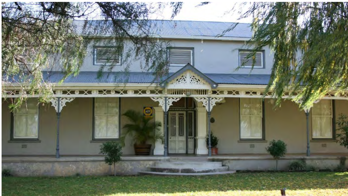
Figure 40. Bethel, front (east) façade (JS 2011).
