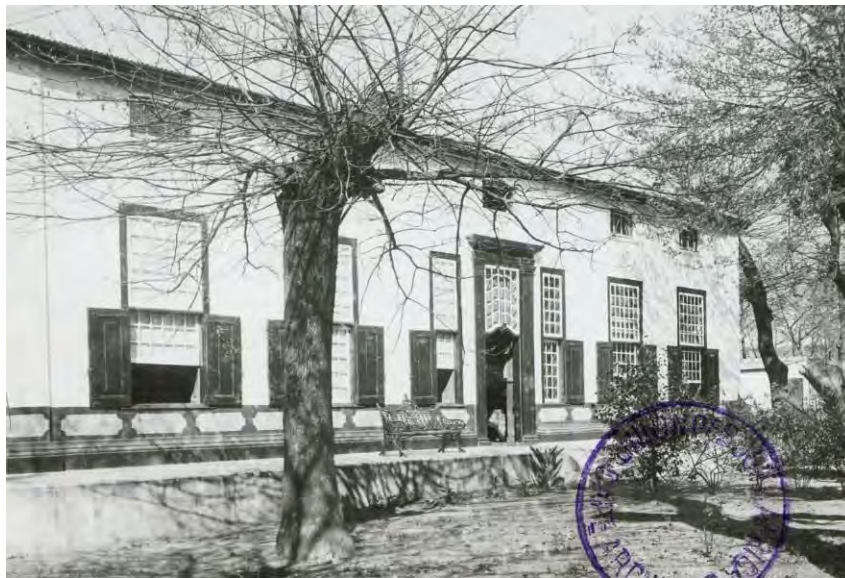
Figure 36. Old Dutch Reformed Parsonage, front (west) façade (Cape Archives).
