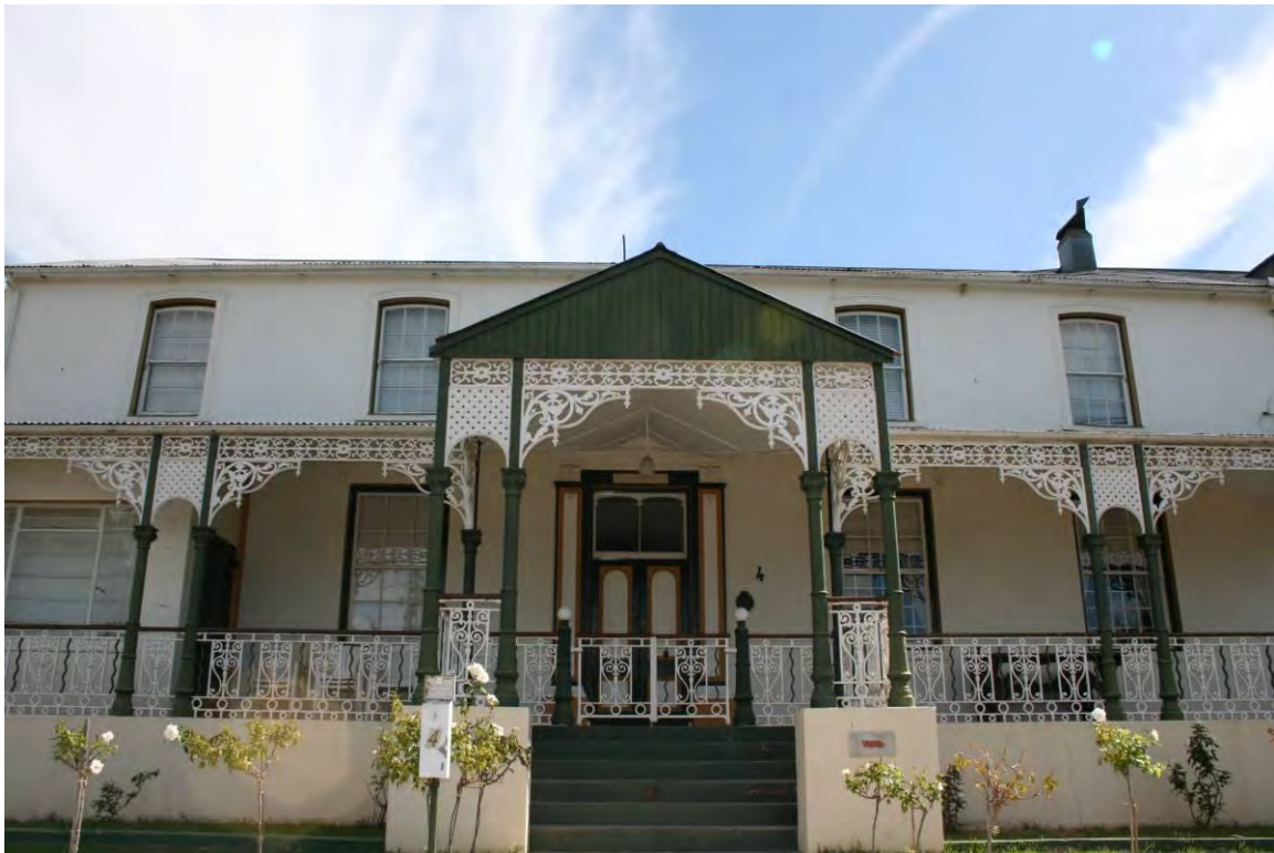
Figure 27. 4 Zeederberg Square, front (east) façade (JS 2011).
