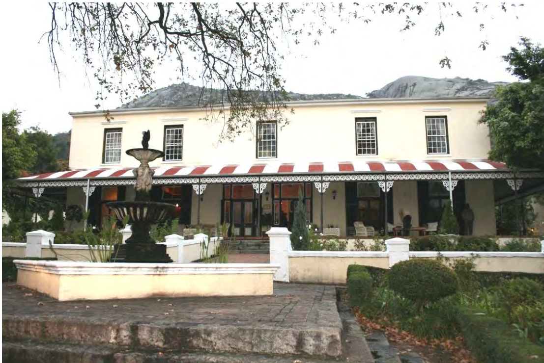
Figure 30. Pontak, front (east) façade (JS 2011).
