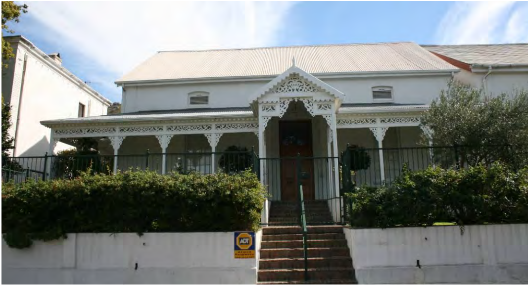
Figure 25. 2 Zeederberg Square, front (east) façade (JS 2011).
