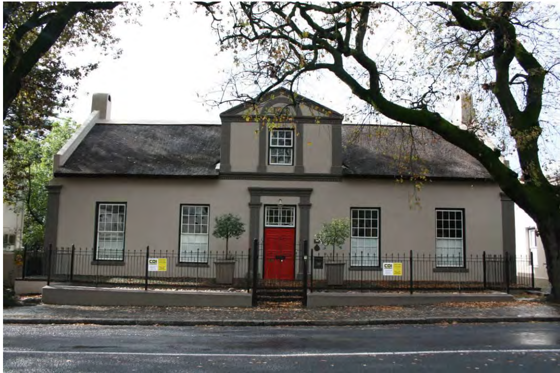
Figure 10. 101 Main Street, front (west) façade (JS 2011).
