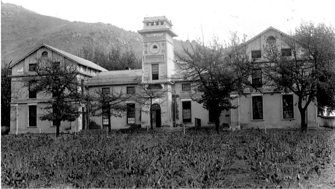
Figure 34. Paarl Gymnasium, front (east) façade (Drakenstein Heemkring HP0021).
