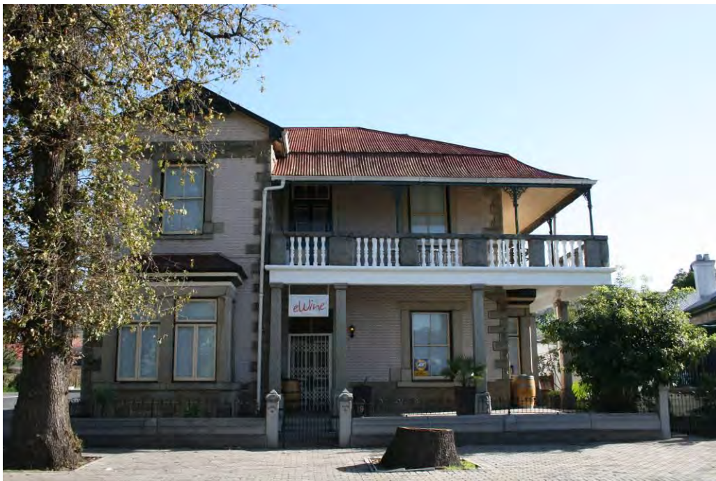
Figure 8. Villa Sarnia, front (east) façade (JS 2011).
