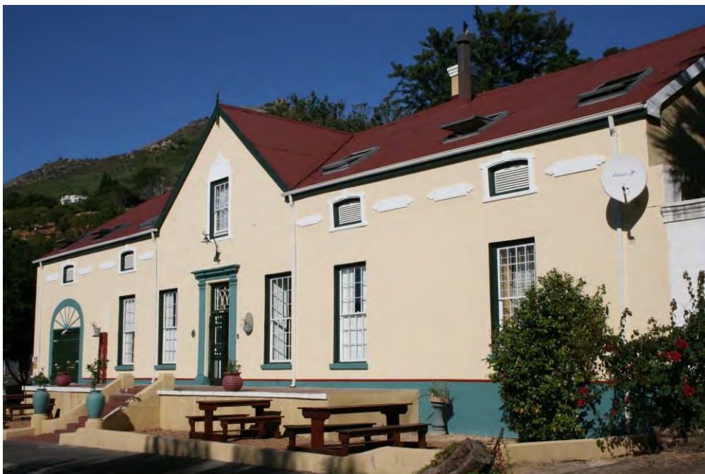
Figure 39. Nantes Vue, front (east) façade (JS 2012).
