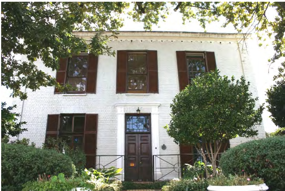
Figure 24. 1 Zeederberg Square, front (east) façade (JS 2011).
