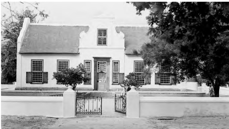
Figure 37. Old Dutch Reformed Parsonage after restoration, front (west) façade (Drakenstein Heemkring).
