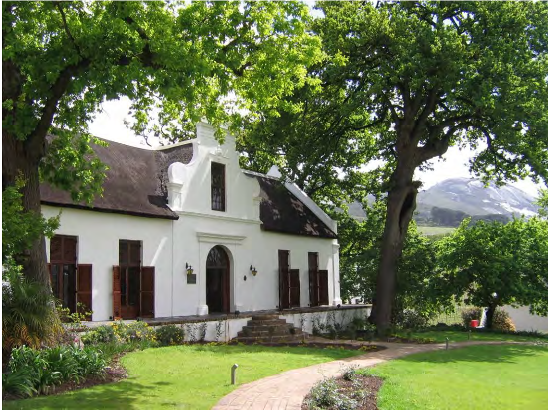
Figure 5. Laborie, front (east) façade (JS 2006).
