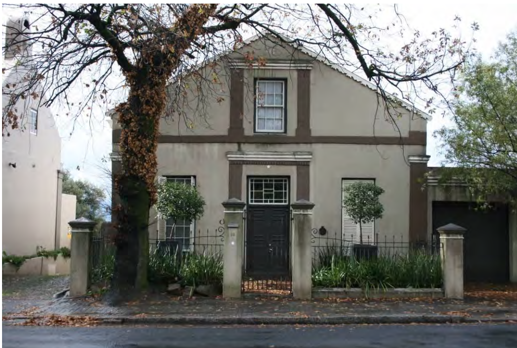
Figure 11. 99 Main Street, front (west) façade (JS 2011).
