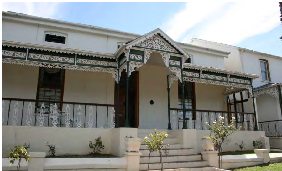
Figure 26. 3 Zeederberg Square, front (east) façade (JS 2011).
