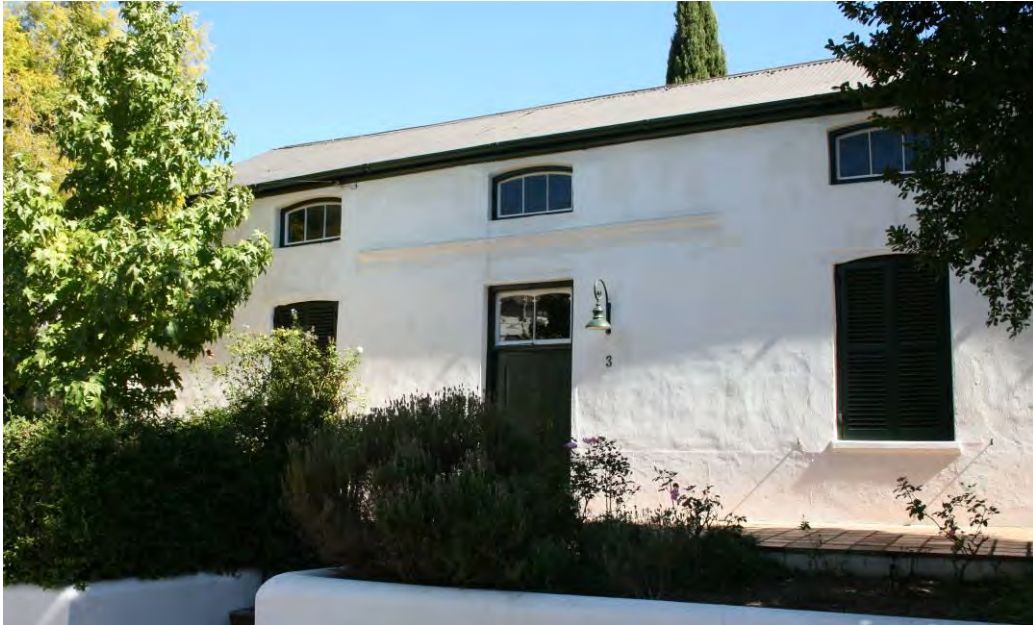
Figure 21. 4 Theron Street, front (east) façade (JS 2011).
