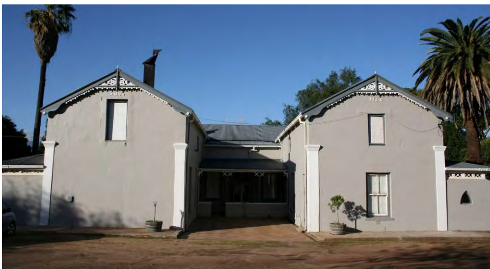
Figure 41. Bethel, back (west) façade (JS 2011).
