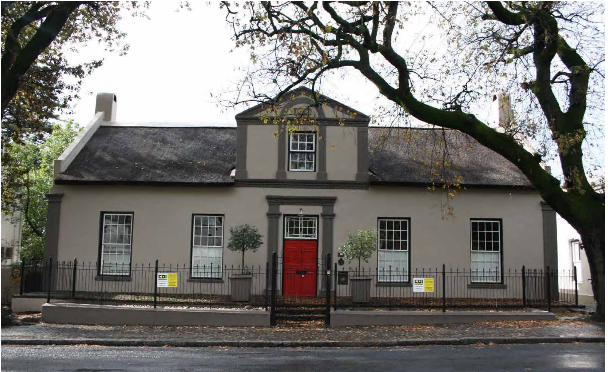
101 Main Street West Facade
